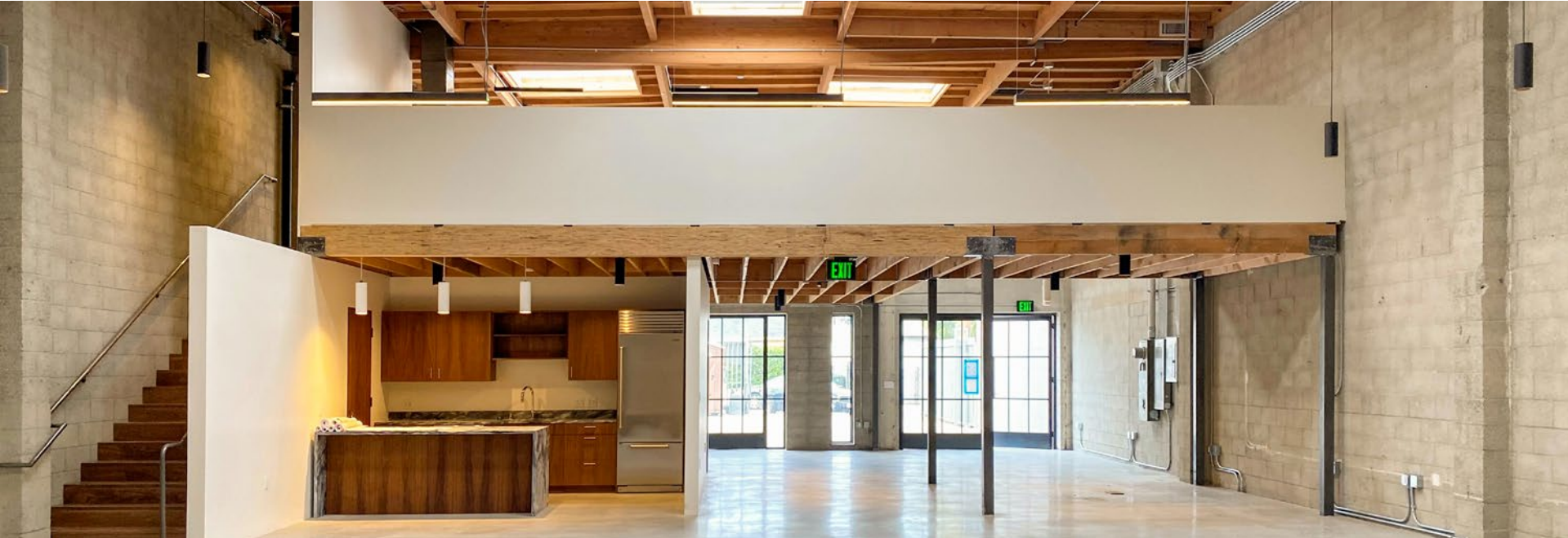
3010 N Coolidge Ave (Under Construction)
