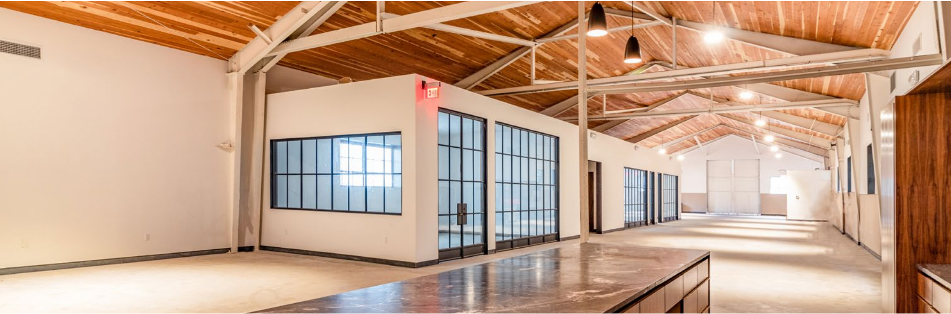
1833 San Fernando Rd (Under Construction)
