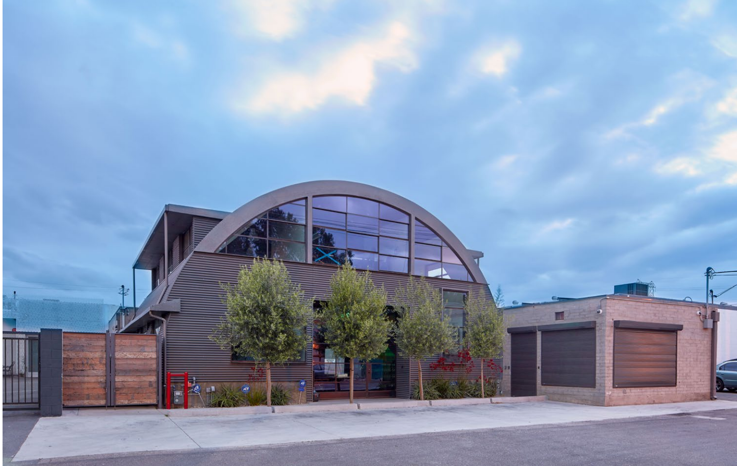
5895 Blackwelder St, post development.
