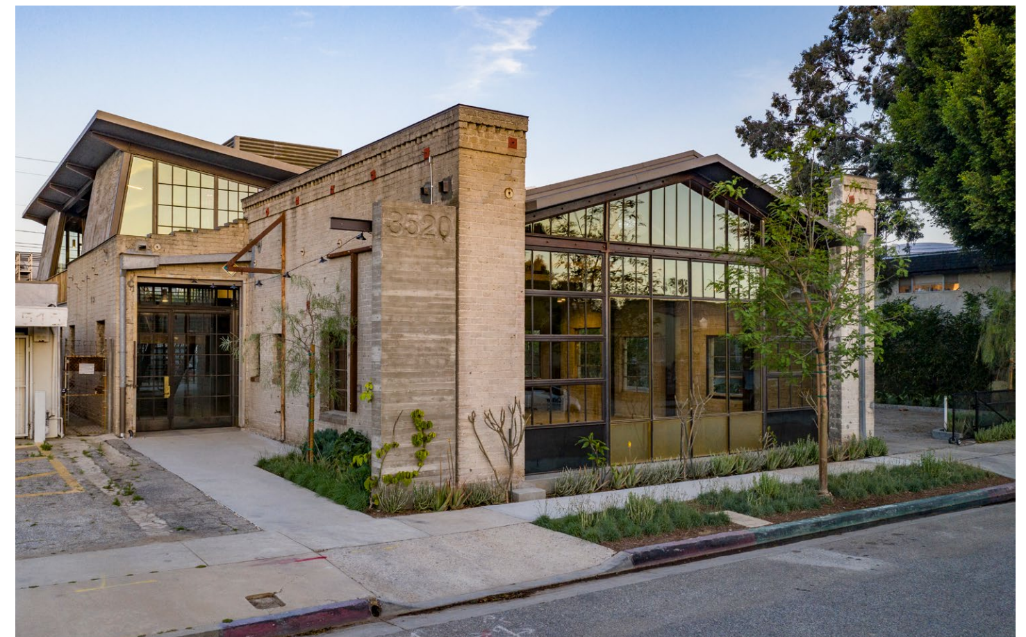
3520-24 Schaefer St, in final construction stage in 2019.
