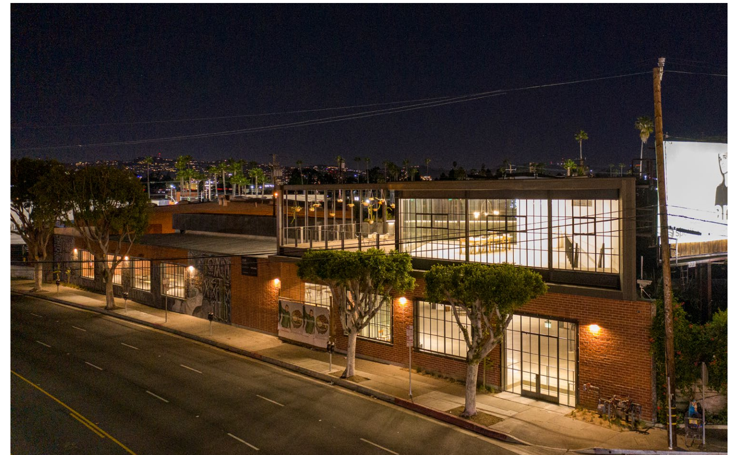
3030 La Cienega Blvd, construction near completion.
