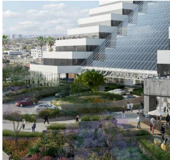
The eight-story building, located on a full block at 10000 Washington Boulevard in Culver City, offers 300,000 square feet of office space on its upper floors and 65,000 square feet of street-level commercial space. Portions of the building have already been leased by WeWork and Equinox Fitness, and Apple is in talks to take the remaining 150,000 SF.
