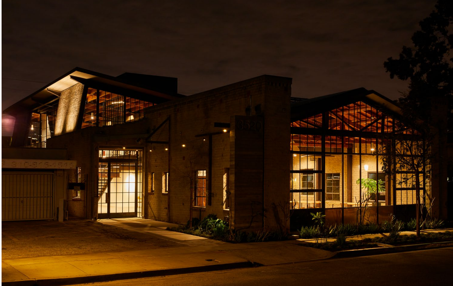
3520-24 Schaefer St, in final construction stage in 2019.
