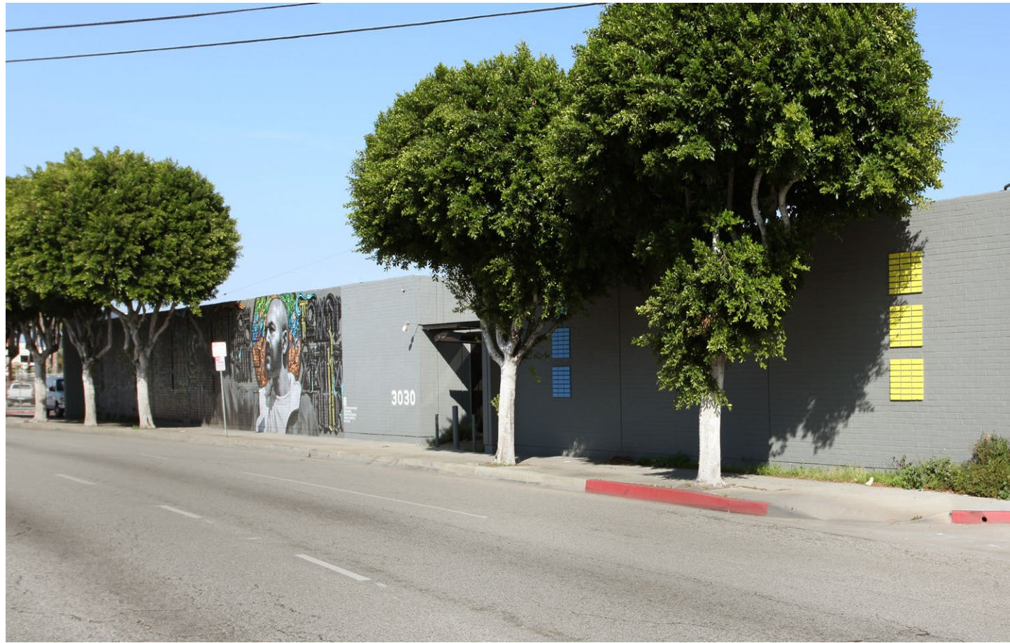
3030 La Cienega Blvd, as acquired in December 2015.
