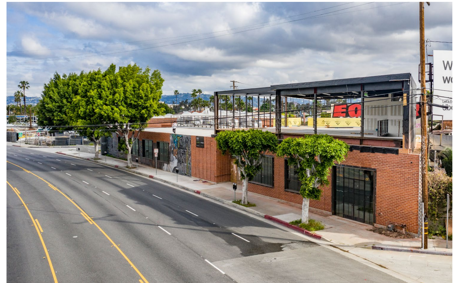
3030 La Cienega Blvd, construction near completion.
