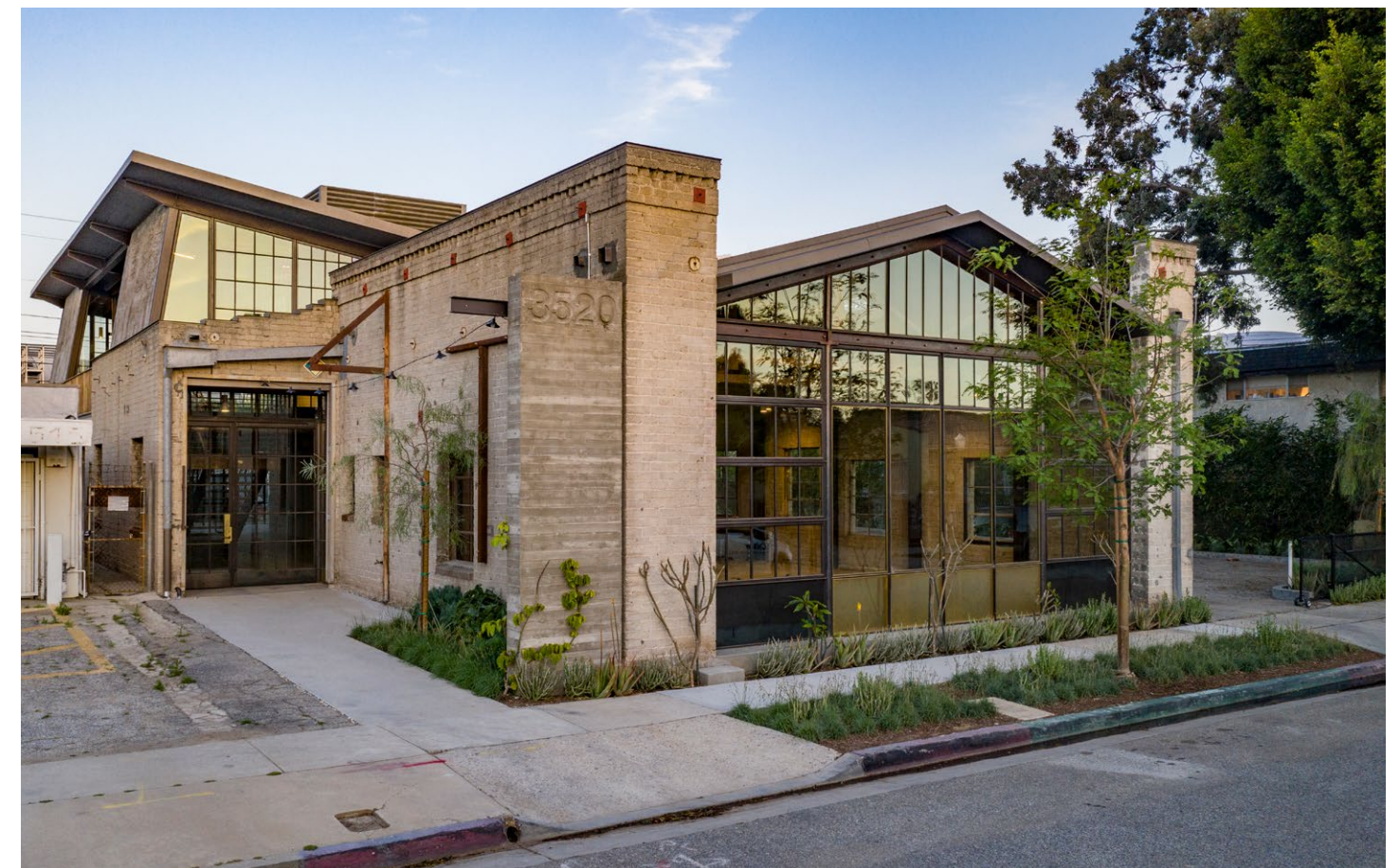
3520-24 Schaefer St, in final construction stage in 2019.
