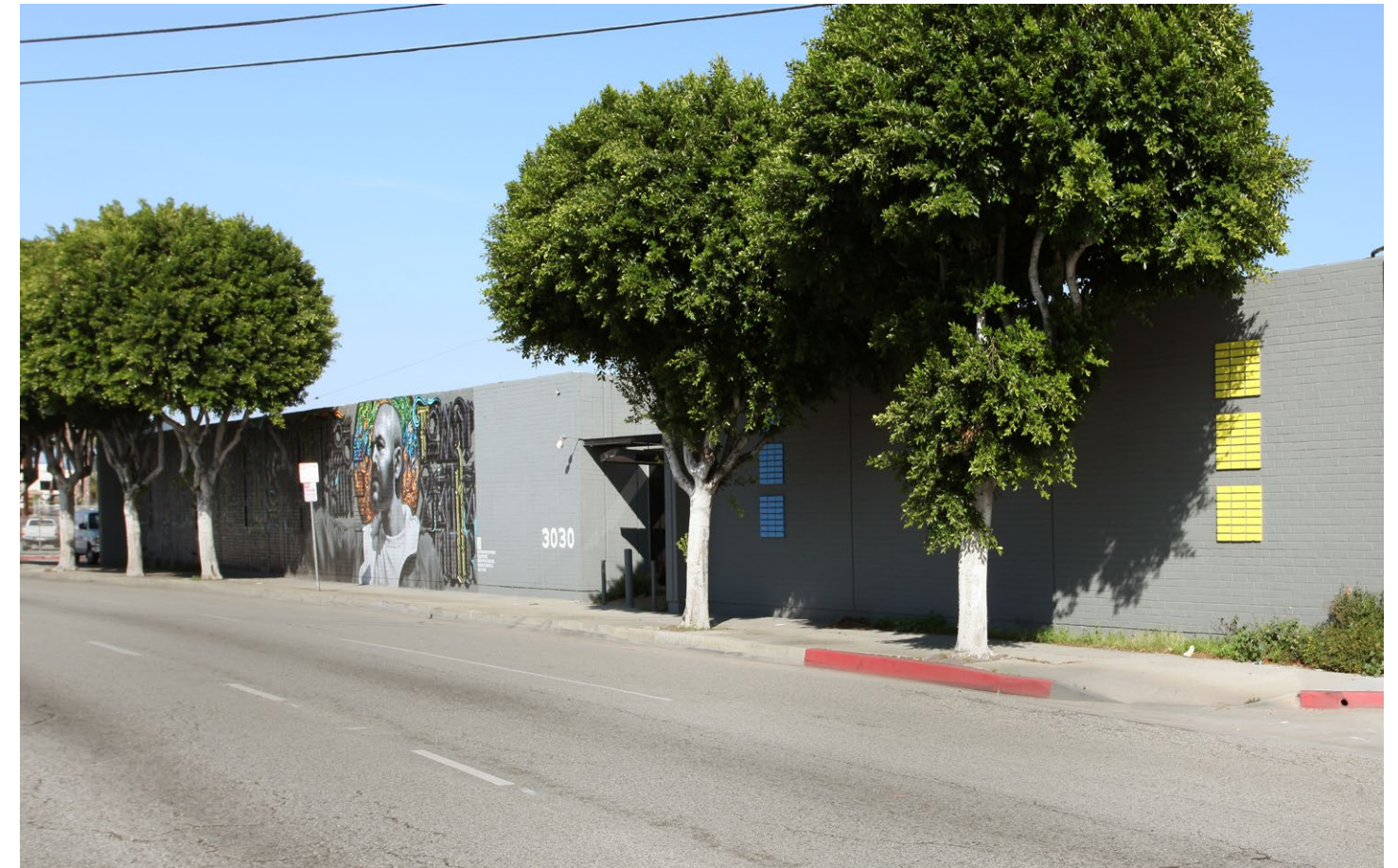
3030 La Cienega Blvd, as acquired in December 2015.
