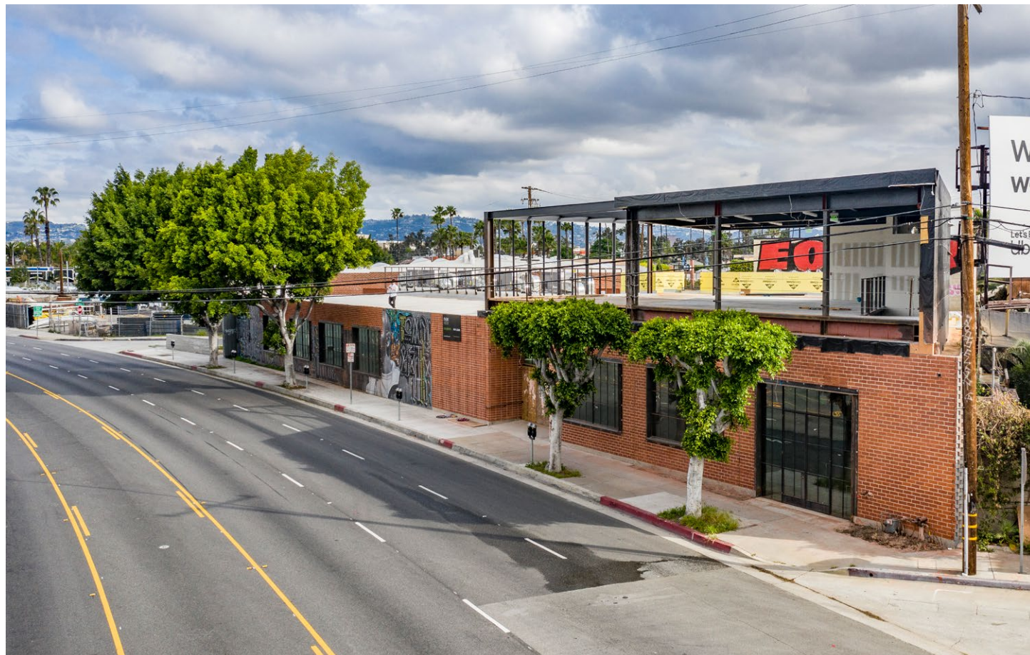
3030 La Cienega Blvd, nearing completion.
