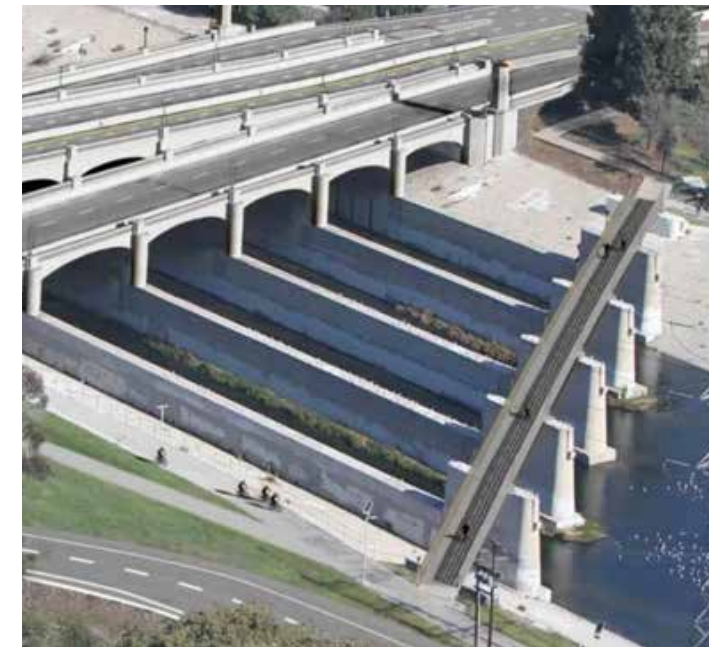
Glendale Hyperion Bridge. Opened in 1928, the bridge will be redesigned and retrofitted for pedestrians, cyclists, and drivers. In addition, an entirely new pedestrian-only bridge will be built just south of the Glendale-Hyperion Viaduct, along a former Pacific Electric Red Car right-of-way, where P.E.'s Glendale-Burbank Line
