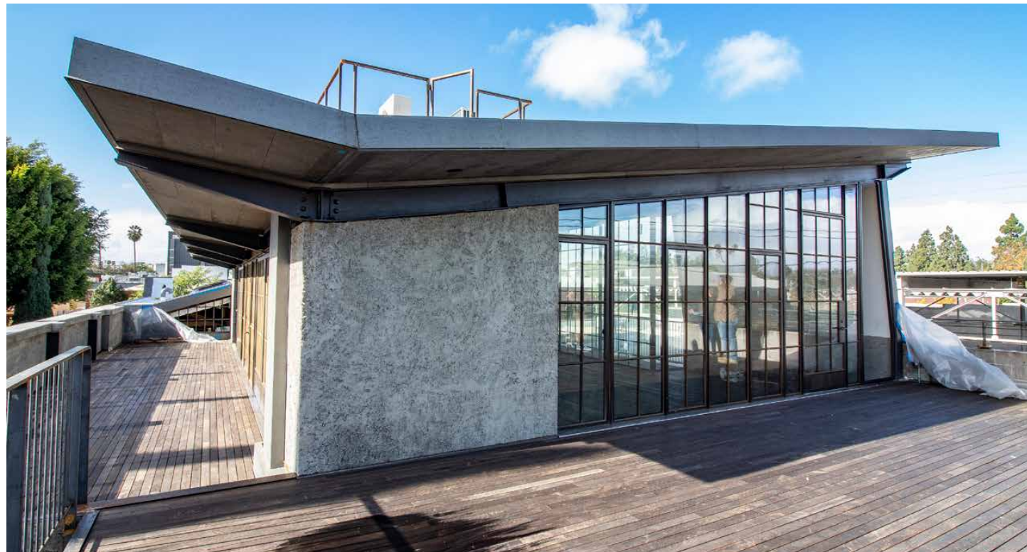
Steel windows, and doors redcar
