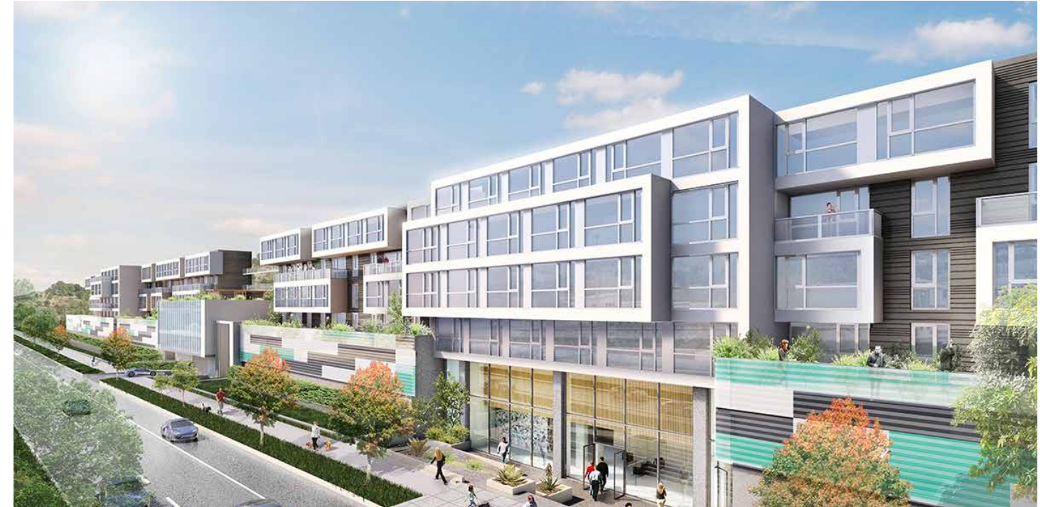
Riverglen II Apartments (C). The development consists of a trio of four-story buildings with one- and two-bedroom dwellings. “Glass-enclosed modules” link the buildings to joint amenities, such as a rooftop pool and a recreation center.
