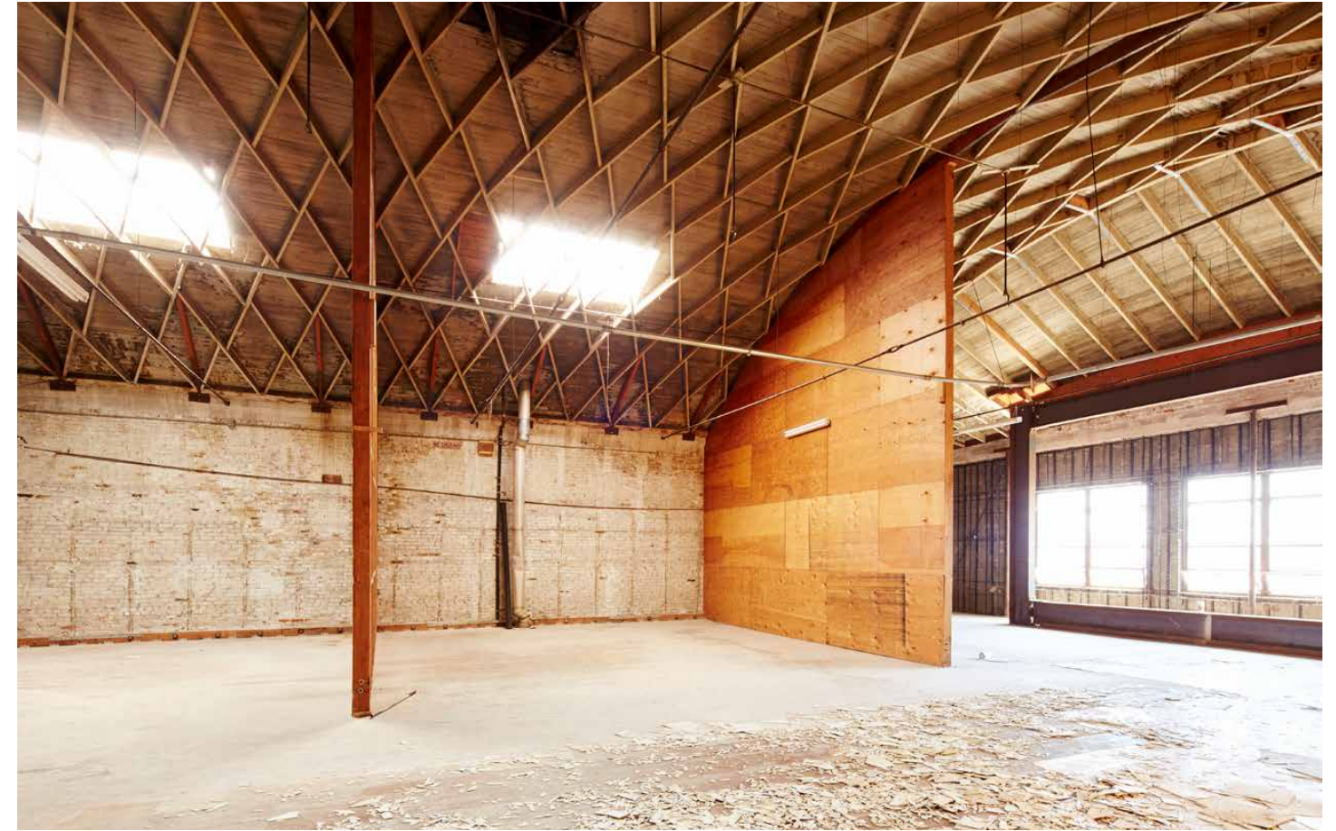
759 N Spring St, during demolition in May 2015.
