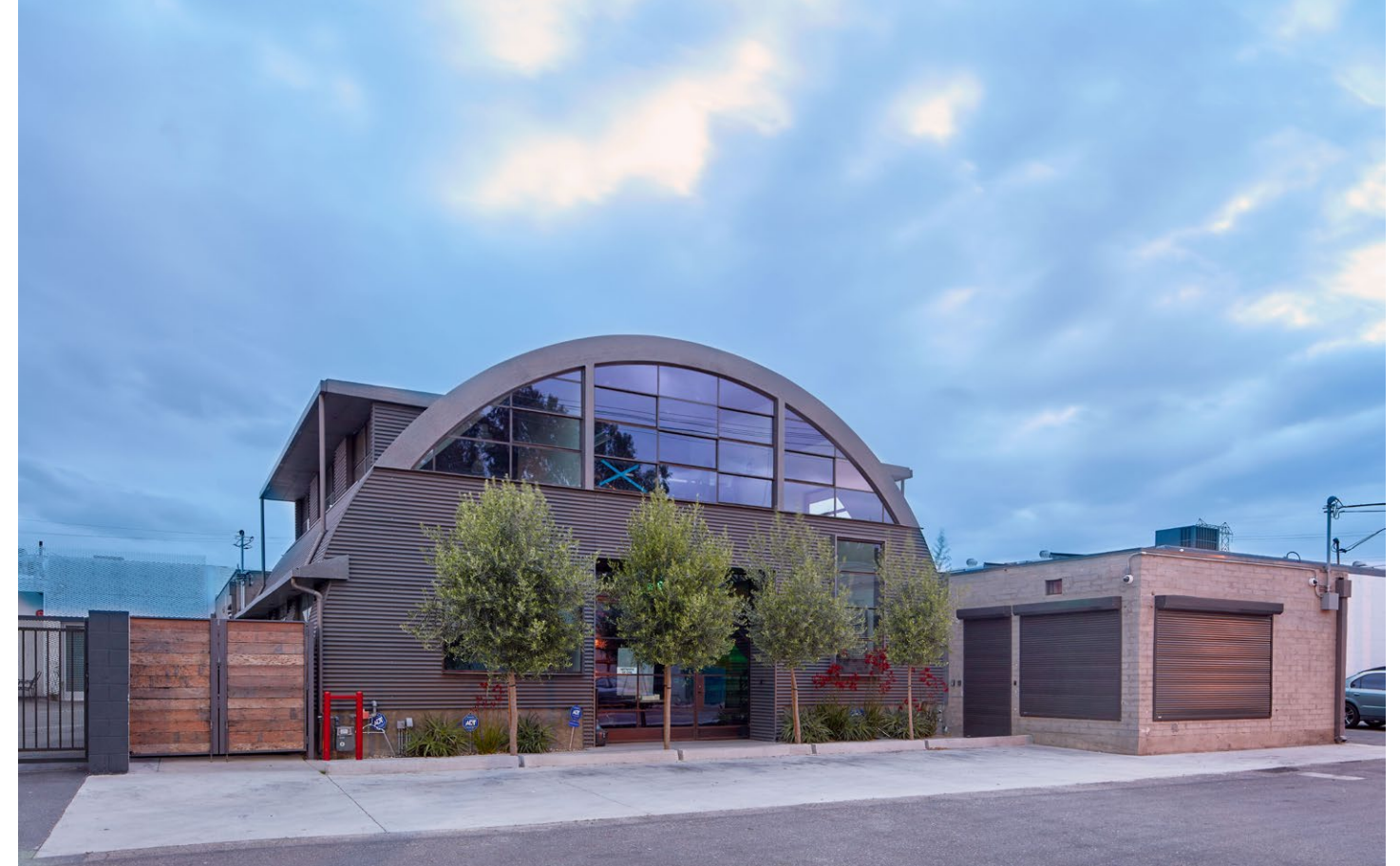
5895 Blackwelder St, post development.
