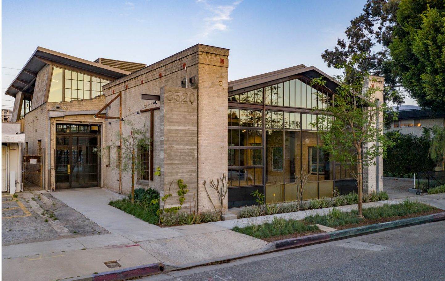
3520-24 Schaefer St, in final construction stage in 2019.
