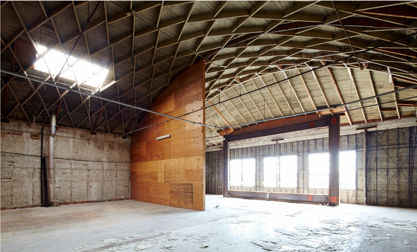
759 N Spring St, during demolition in May 2015.
