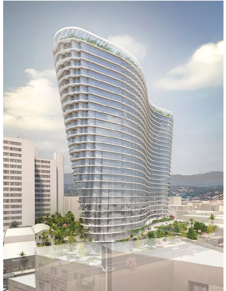
Redcar recently sold 643-675 N Spring St to French real estate investment company Compagnie de Phalsbourg. Development plans call for 300 apartments, 149 hotel rooms, shops, and public open space. Design comes from award-winning architecture firm Studio Gang.
