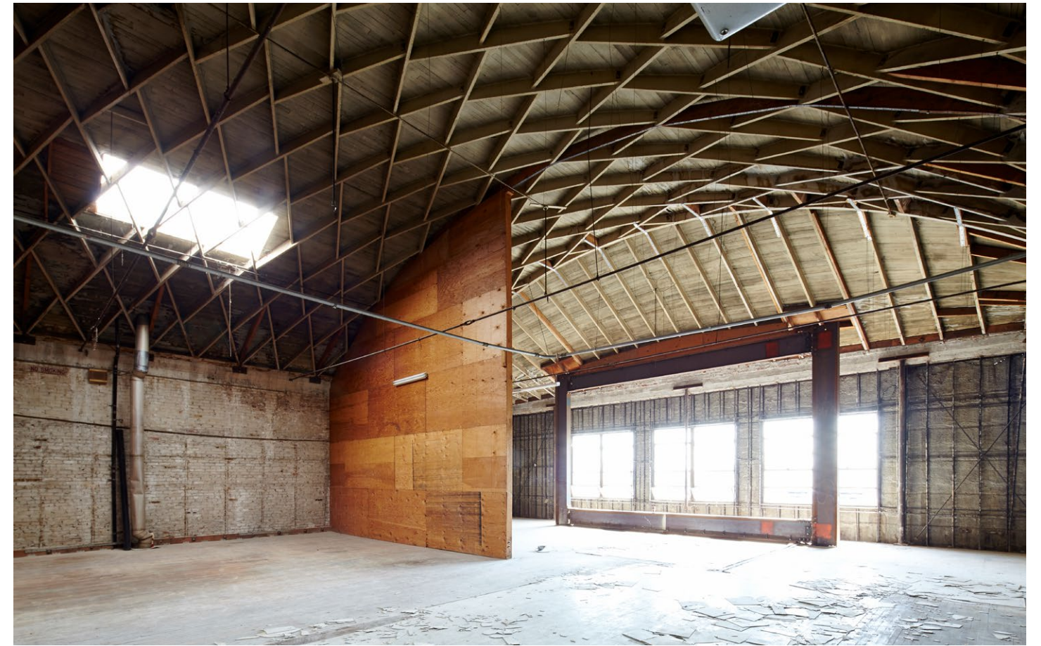
759 N Spring St, during demolition in May 2015.
