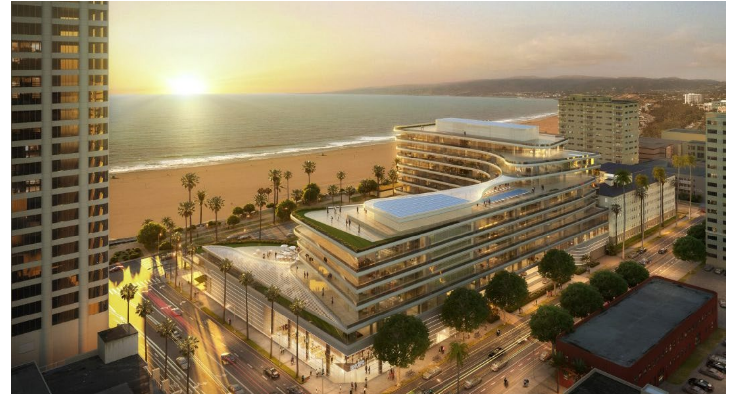
The Miramar Santa Monica (G). The project, located at the terminus of Wilshire Boulevard, now calls for 312 guest rooms, a maximum of 60 market-rate condominiums, 475 basement parking spaces, and a 100 percent affordable housing building at 1127 2nd Street. Over half of the total property will remain as open space, including 14,000 square feet of publicly-accessible gardens.
